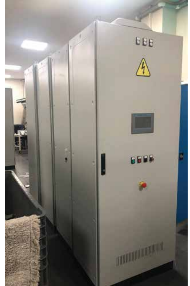
Mobile Units Sewage Treatment Project For Construction Camps North-Africa 2020
