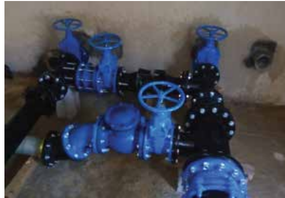
Water Network Project Lebanon 2017
