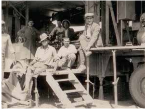
Pipeline Project Iraq 1932
