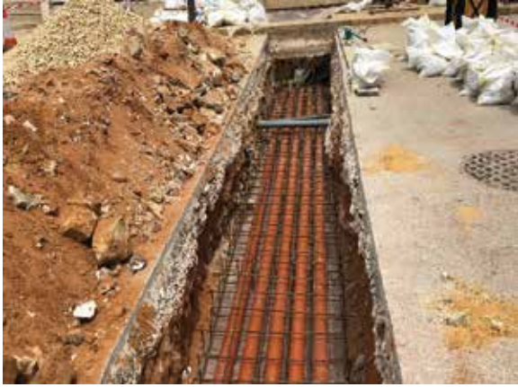
Water Network Project Lebanon 2015
