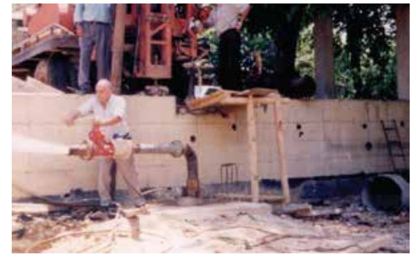
Greater Beirut Water Infrastructure Project Lebanon 1999
