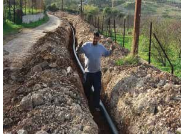
Water Network Project Lebanon 2017
