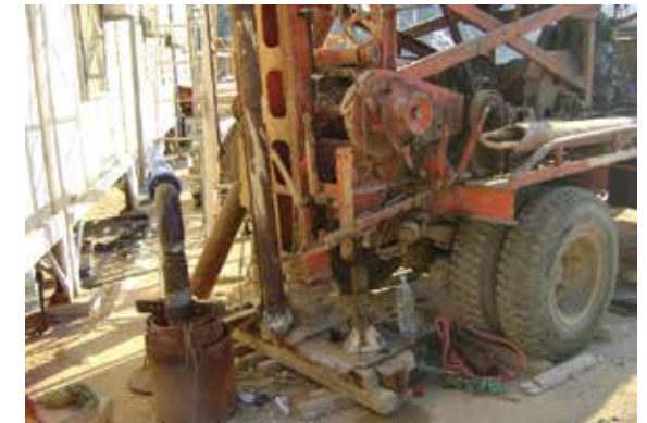
700 CM/Hr Sea Water Intake Wells For SWRO Plant Lebanon 2015
